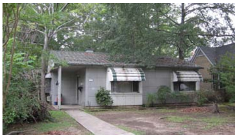
At 1302 Tyler Street is a Lustron House which was built with an exterior of steel porcelain panels.
