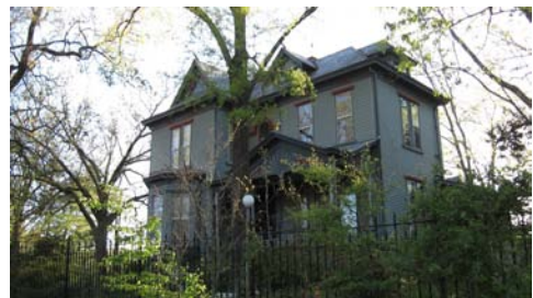
Queen Anne style dwelling at 2122 S. Scott Street.
