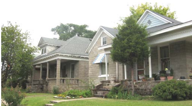
The Hanger Hill Historic District contains numerous dwellings built of concrete block.
