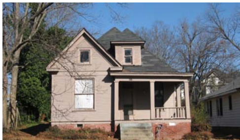
Thousands of notable properties built before 1945 remain to be inventoried and evaluated in areas such as the Stephens Neighborhood (3410 W. 13 th Street).
