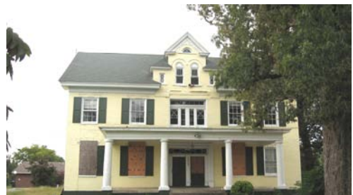
The Woodruff House is a notable example of the Colonial Revival style, but is currently vacant at 1017 E. 8 th Street.
