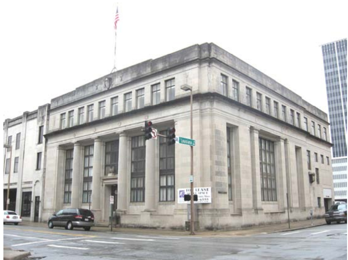
A downtown survey would identify properties listed on the National Register, their condition and available space for rehabilitation (Federal Reserve Bank, 123 W. Third Street).
