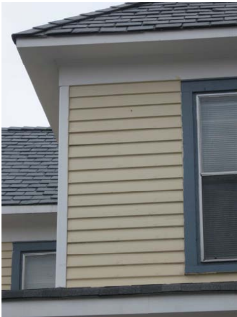
Dwellings built in the early 20 th century were built with old-growth lumber which is now expensive and difficult to obtain.
