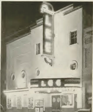
Below—Daytime appearance of the old Highland at Little Rock, Ark., before it was demolished to make way for its modern successor, the new Lee Theatre, shown in formal evening dress at the right. A convincing argument for property renovation.
