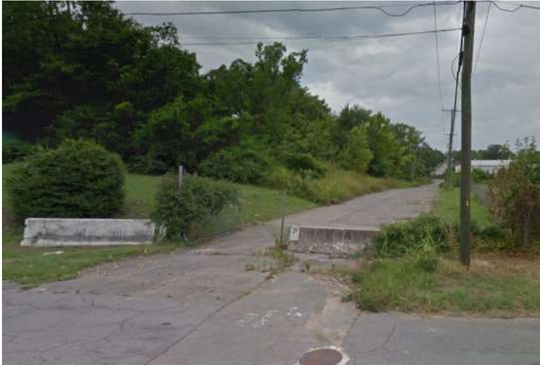
Figure 58 – Connection #7. The access point to the Corridor at 10 th is almost complete already.
