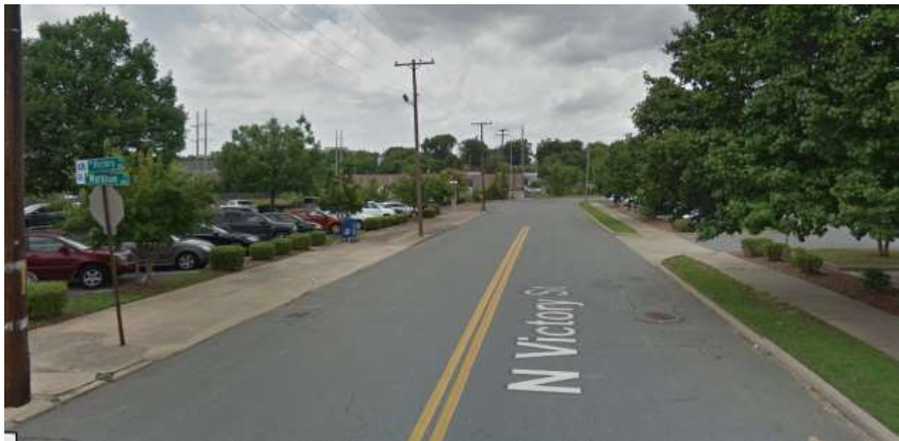
Figure 22. Google streetview of N. Victory St. from the corner of N. Victory and Markham. The street is 36' wide, has a low average daily traffic count, and the sidewalk on the west side is in good repair.
