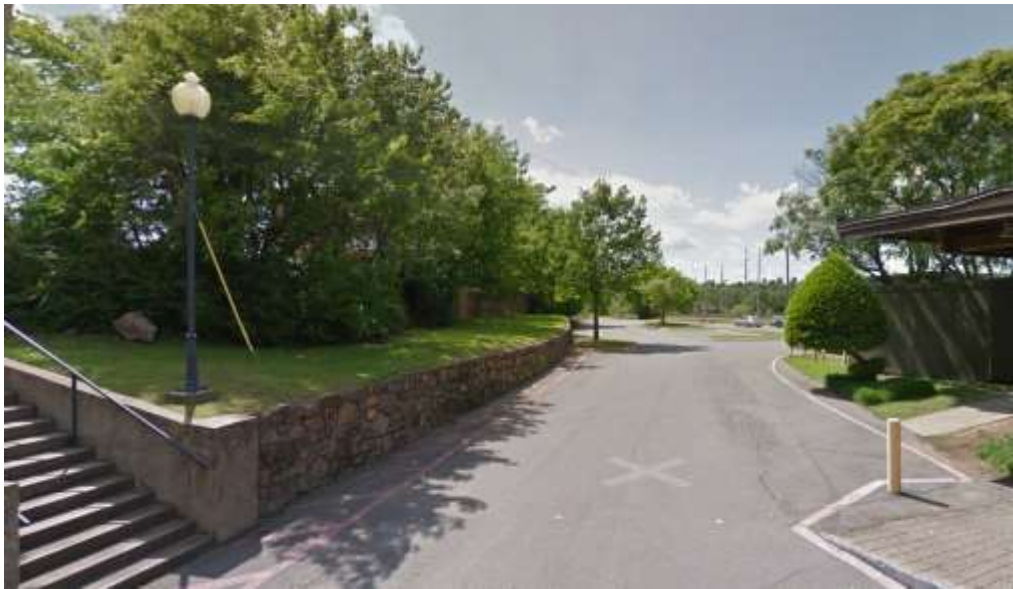
Figure 32. Instead of running the trail along the southern wall, immediately after the stairway (bottom left), a portion of the wall could be removed and the trail could ramp up to the greenspace in between the two walls. Construction would cost more but the south wall parking spots would be retained. The area between the two walls is approximately 18'. We would have to survey this area to see if there is adequate ROW. If this was the Corridor route, we may want to erect a fence along the lower wall to prevent falls. Note too the challenge the ramp on the bottom right will create to creating the trail. Mark Webre suggested that the stairway could be moved to facilitate separation between vehicles and BikePed traffic in this narrow area.
