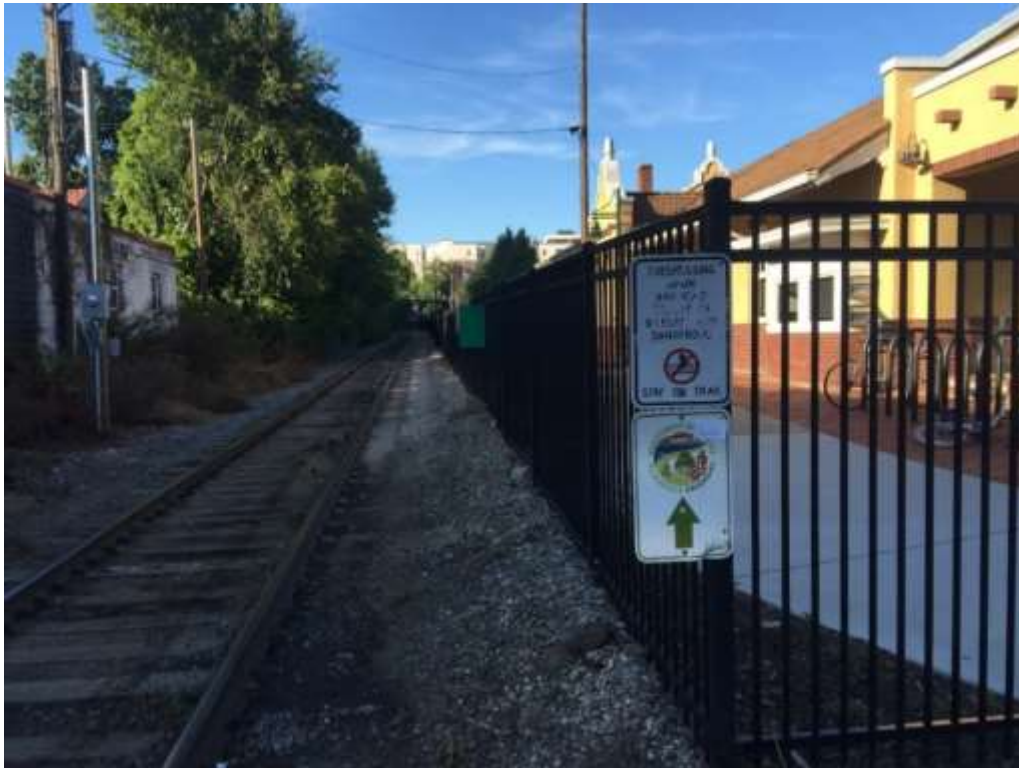
Figure 3. The setback between the Razorback Greenway and active railroad tracks is approximately six feet at its intersection with Dickson St. Photo courtesy of Mandy Bunch.
