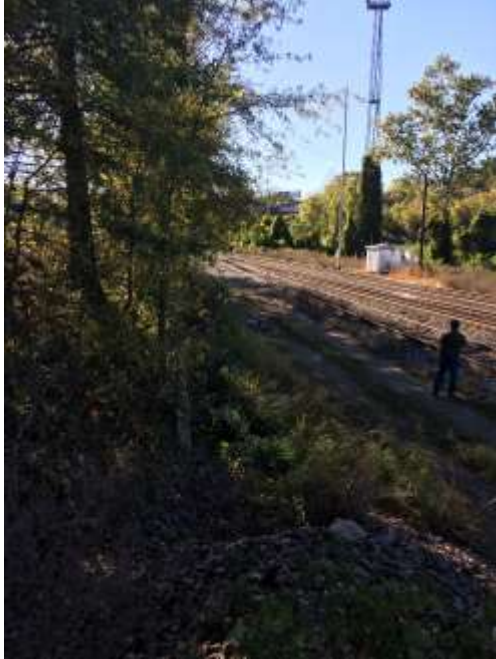
Figure 34. The slope the Corridor would travel along and up to meet 2 nd St. What is not easily seen in this photo is that the difference in elevation between 2 nd St. and the tracks is decreasing as distance from the camera increases. The Corridor would run parallel to 2 nd St., meeting it at around 270 ft. above sea level. This 8 ft. rise in elevation over ~250 ft. would create a ~3.2% grade on the Corridor (well within minimum standards), and the retaining wall required would create separation from the Union Pacific tracks and thereby increase safety. Leland Couch pictured for scale.
