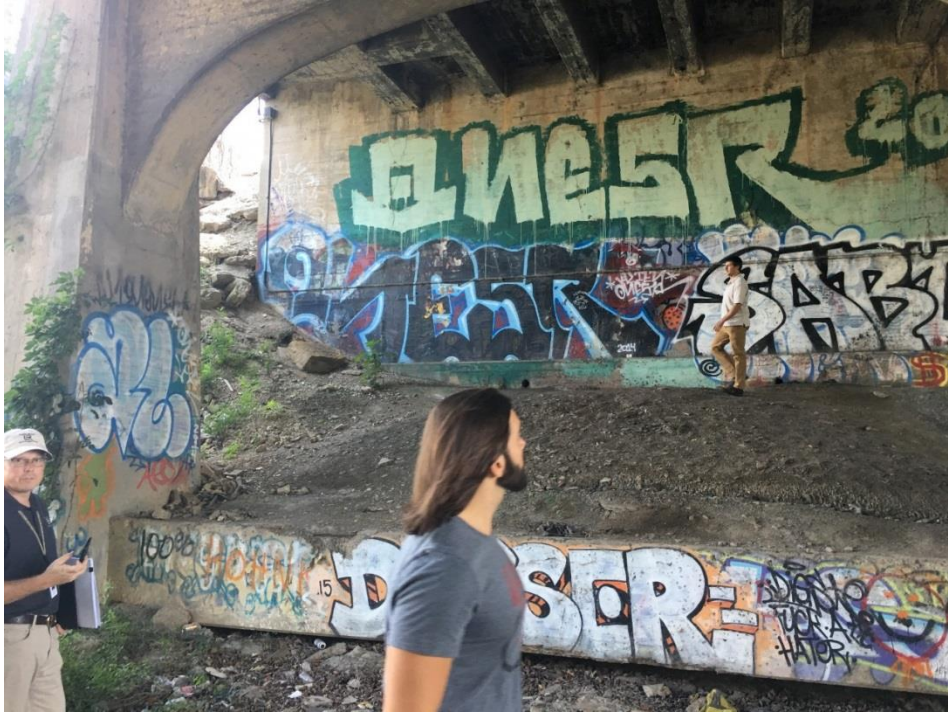
Figure 7. We will extend the 3 ft. wall associated with the pillars approximately 7 ft. higher to create a level platform for the trail approximately 10 ft. higher than the grade of the tracks. The man standing at the top of the picture is approximately standing at the trail's proposed grade.
