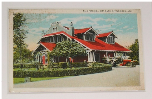
Figure 3. Historic postcard of Fire Station #2 at 1201 Commerce Street.
