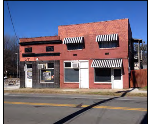
Figure 38. Commercial node on 9th Street
