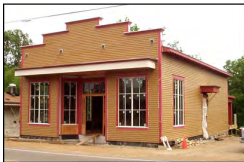
Figure 81. Clapboard siding would be an acceptable cladding for a new commercial building in the district. However, since brick is the more dominant cladding for this building type, brick should continue to be the primary material for most new commercial and mixed-use buildings in MacArthur Park.
