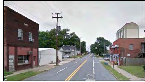
Figure 73. This small node of older commercial buildings on E. 9 th Street is perhaps the only intact grouping of such buildings in the district. Concerns with insuring that new non-residential buildings in this area are compatible should be stronger here than elsewhere within the district.
