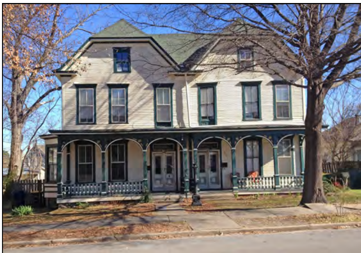
Figure 125. Gemmil House, 1415-1417 Cumberland Street
