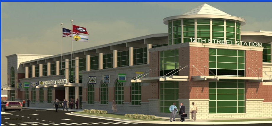
12th Street Sub Station
