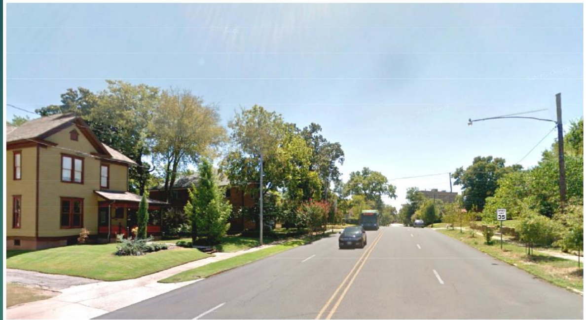
1400 Block – existing 4 lanes
