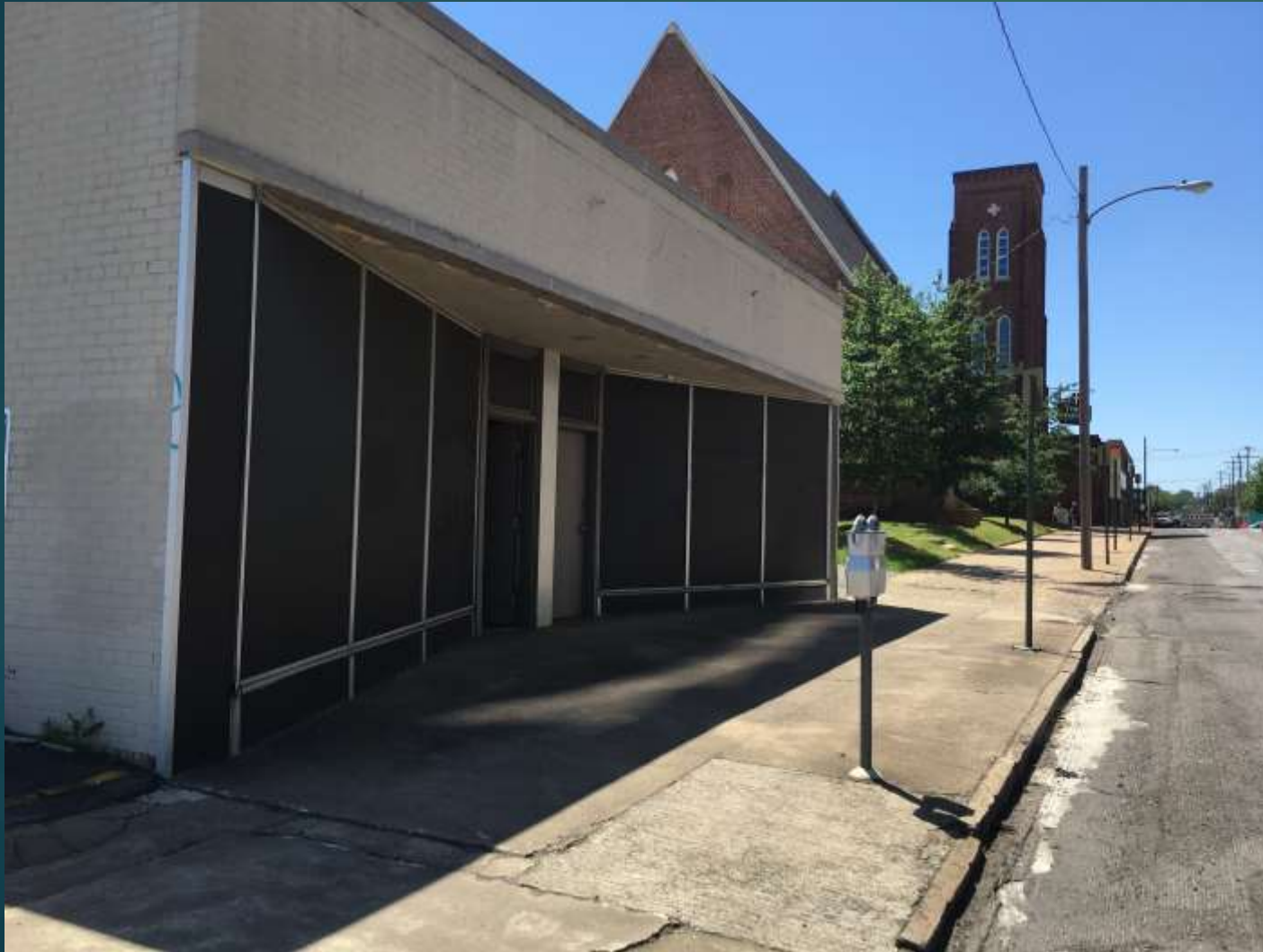
Vacant storefront between Gaines and Arch.
