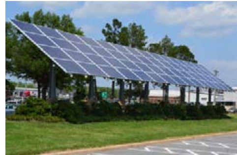
Solar panels at L’Oreal in North Little Rock.
