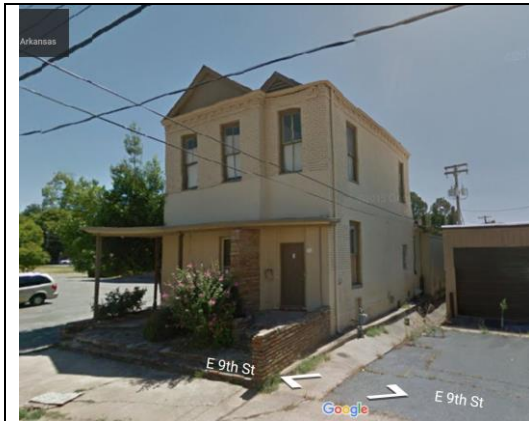
Google Street view of north and west elevation
