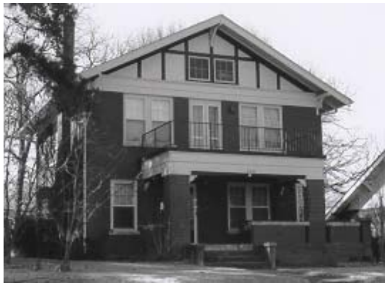
This structure at 108 Thayer reflects the American Foursquare style of construction, in this case embellished with English Revival-style details. AHPP photo.
