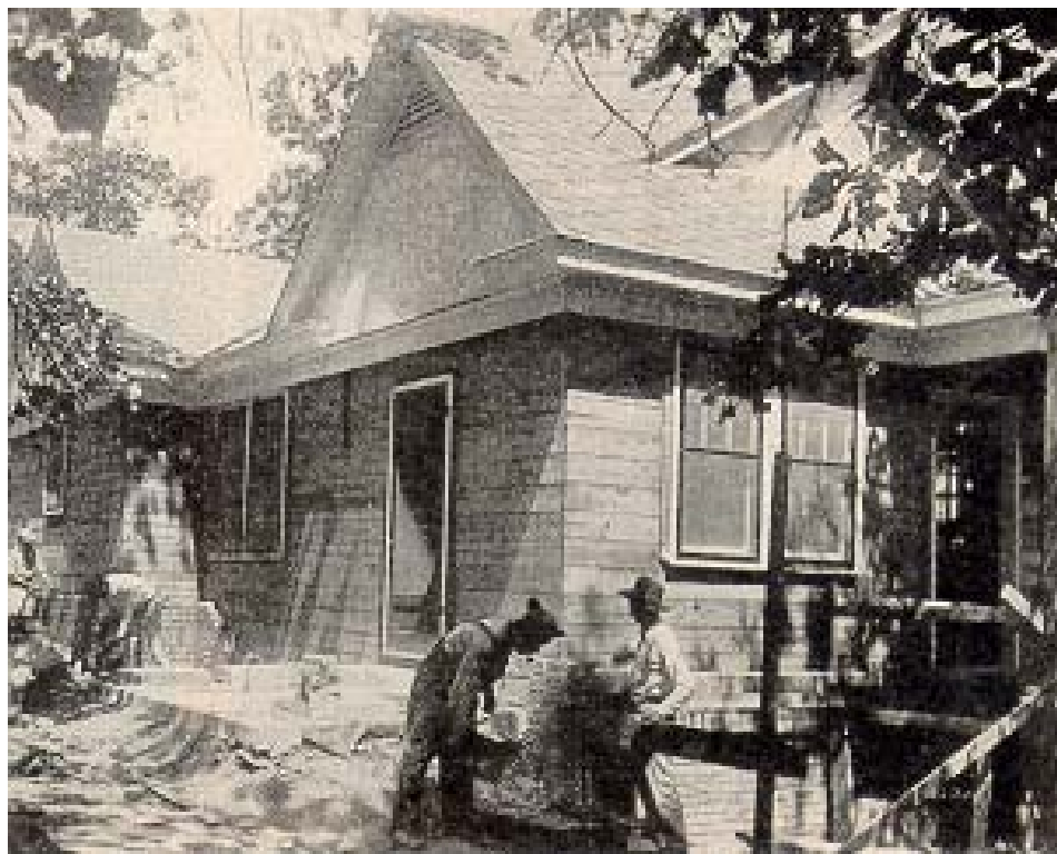
Masons apply brick to house in Capitol View Neighborhood, 1928.
