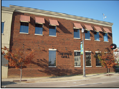
The front façade of this new building lacks a front entrance to address the street. Such a design may be inappropriate in the MacArthur Park Historic District.
