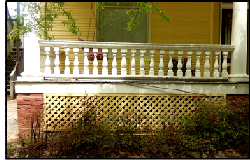
This front porch on 15 th Street has many of the design features found throughout the district: brick piers, lattice work between the piers, and well-proportioned posts, hand railing and balustrade.
