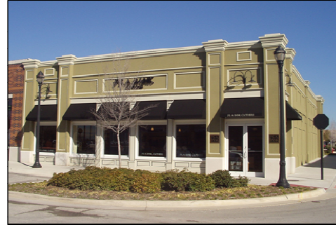
This new infill commercial building has many of the characteristics consistent with these design guidelines, including: front setback on the street ROW, a flat roof screened with a parapet wall, the use of pilasters to break up the façade into vertical bays, paneled wood bulkheads, transoms, awnings, and a well-defined primary entrance off the associated street.
