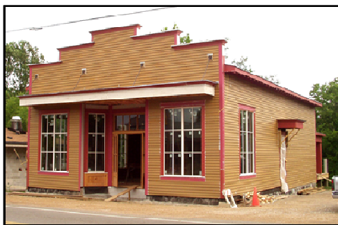
Clapboard siding would be an acceptable cladding for a new commercial building in the district. However, since brick is the more dominant cladding for this building type, brick should continue to be the primary material for most new commercial and mixed-use buildings in MacArthur Park.
