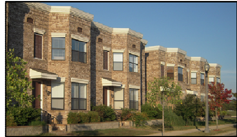
These new townhouses have utilized corniced parapet walls to visually screen their flat roofs.
