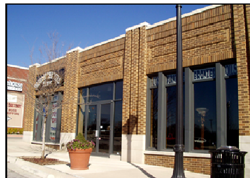
This new building uses pilasters to break up the massing of its façade.
