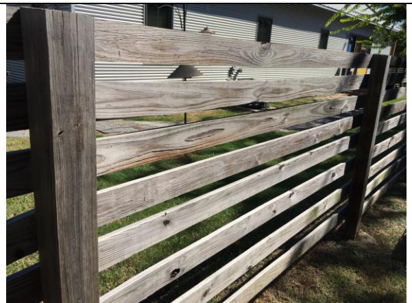
Detail of existing fence.
