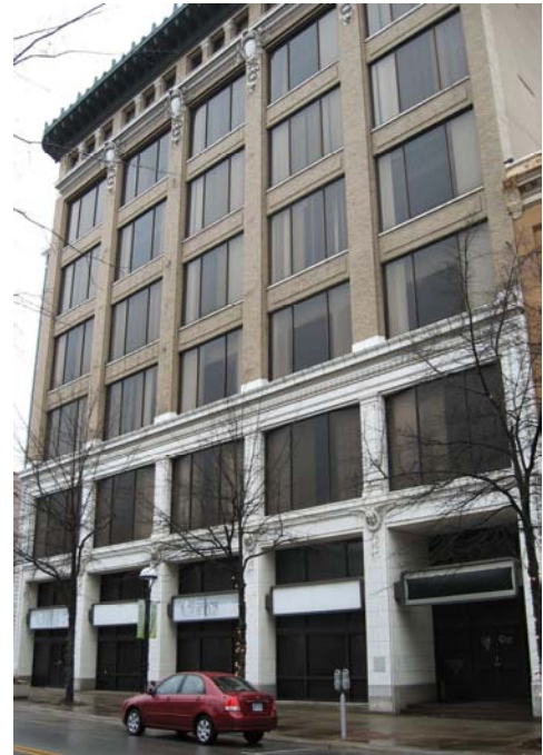
The National Register-listed Gus Blass Department Store at 320-322 S. Main Street would qualify for the federal rehabilitation tax credit.
