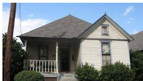
A Conservation Zoning overlay in historic districts such as Marshall Square would require design review only for additions to houses but not for siding, window or porch alterations (802 E. 18 th Street).
