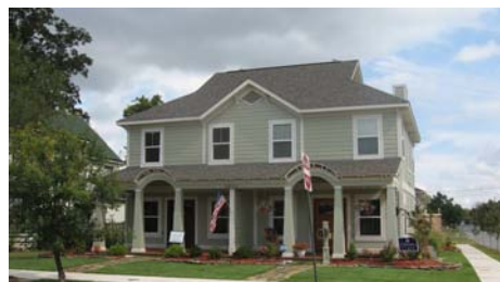
Conservation zoning or limited historic ordinance districts would ensure that new construction was compatible with adjacent historic buildings. This new dwelling was subject to design review in the MacArthur Park Historic District (1421 Cumberland Street).
