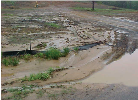
Uncontrolled storm water run off from a construction site.
