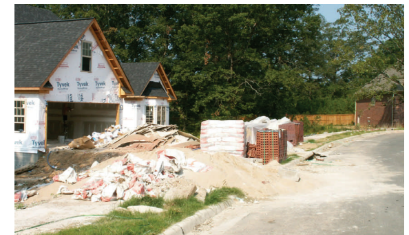
Example of a poorly maintained construction site. Note the sand piled into the street and un-contained debris and trash.
