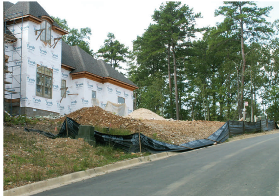
This silt fence is not being maintained properly. It should be re-installed to contain storm water run off.
