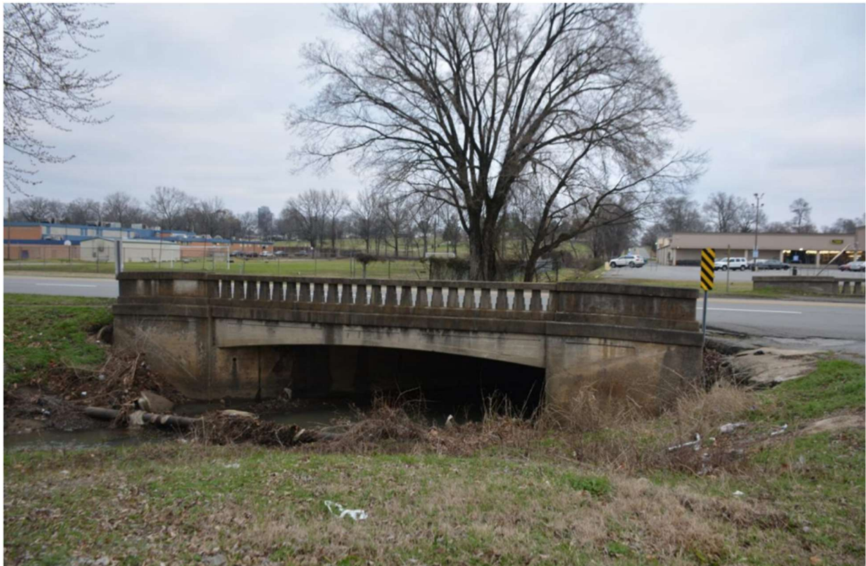
Figure 1. Roosevelt Road Bridge, Photo by AHPP staff, 2025.
