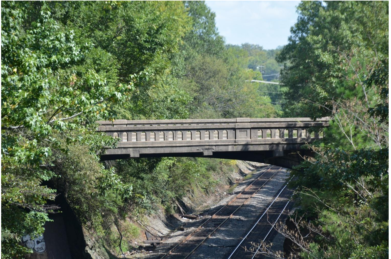
Figure 7: West 12 th Street Overpass, Little Rock, 2024. Photo from the files of the Arkansas Historic Preservation Program.
