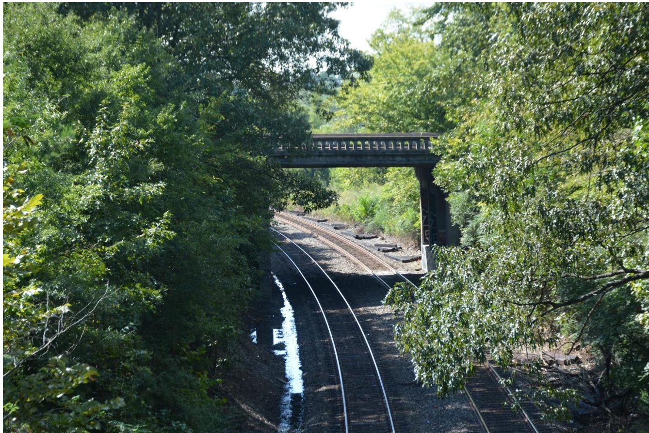
Figure 8: West 14 th Street Overpass, Little Rock, 2024. Photo from the files of the Arkansas Historic Preservation Program.
