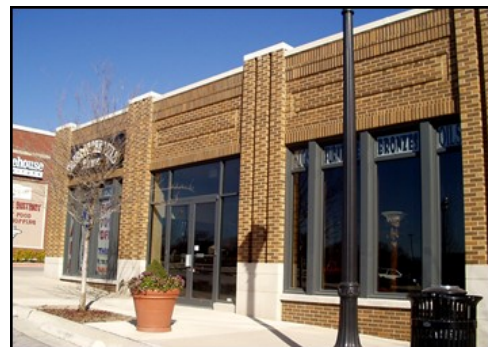
Figure 79. This new building uses pilasters to break up the massing of its façade.
