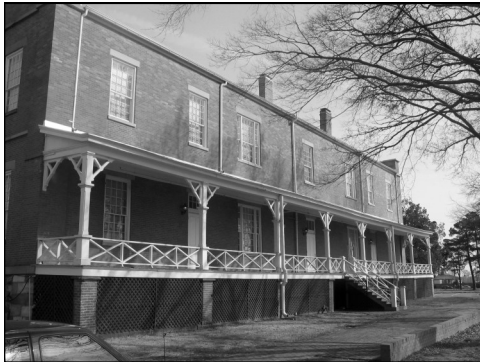
Figure 107 The Arsenal Building (south elevation)
