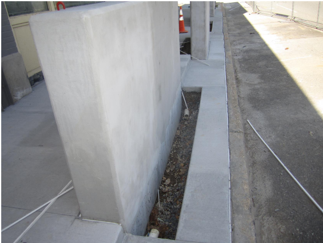
CONCRETE PLANTERS @ THE NORTH SIDEWALK
