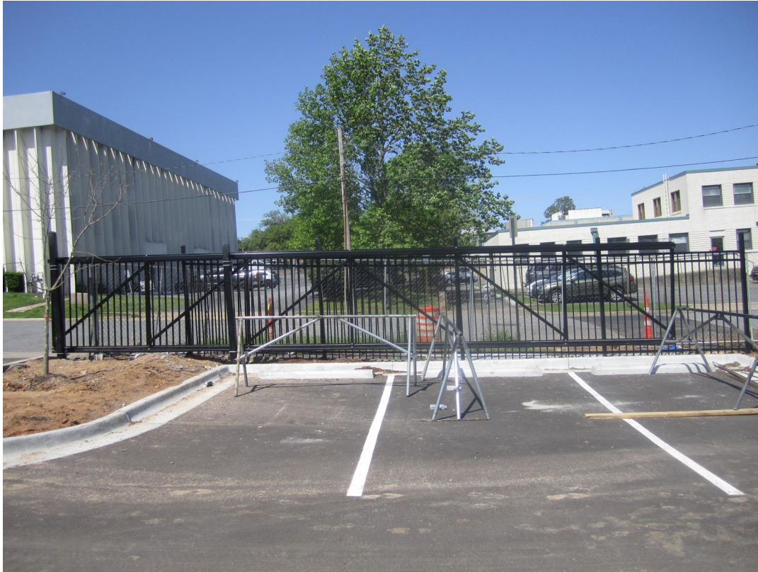
ROLLING GATES AND PERIMETER FENCING HAS BEEN INSTALLED
