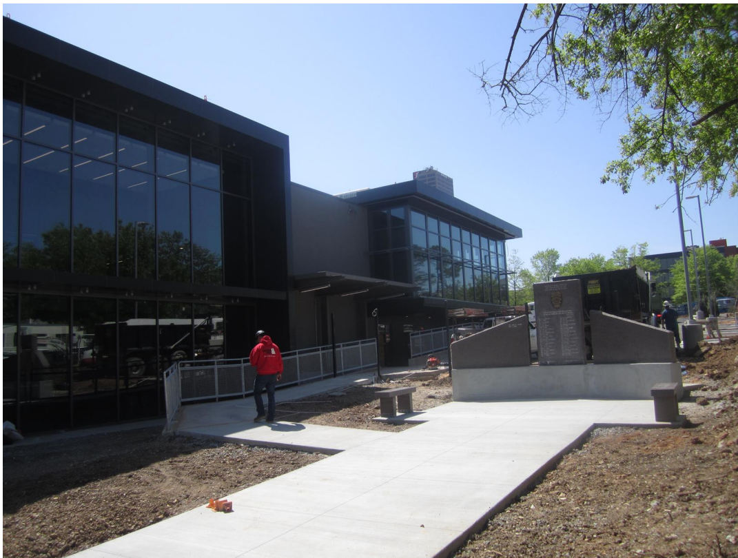
MEMORIAL WALL HAS BEEN INSTALLED ON TO THE NEW CONCRETE BASE ALONG WITH THE NEW PLAZA
