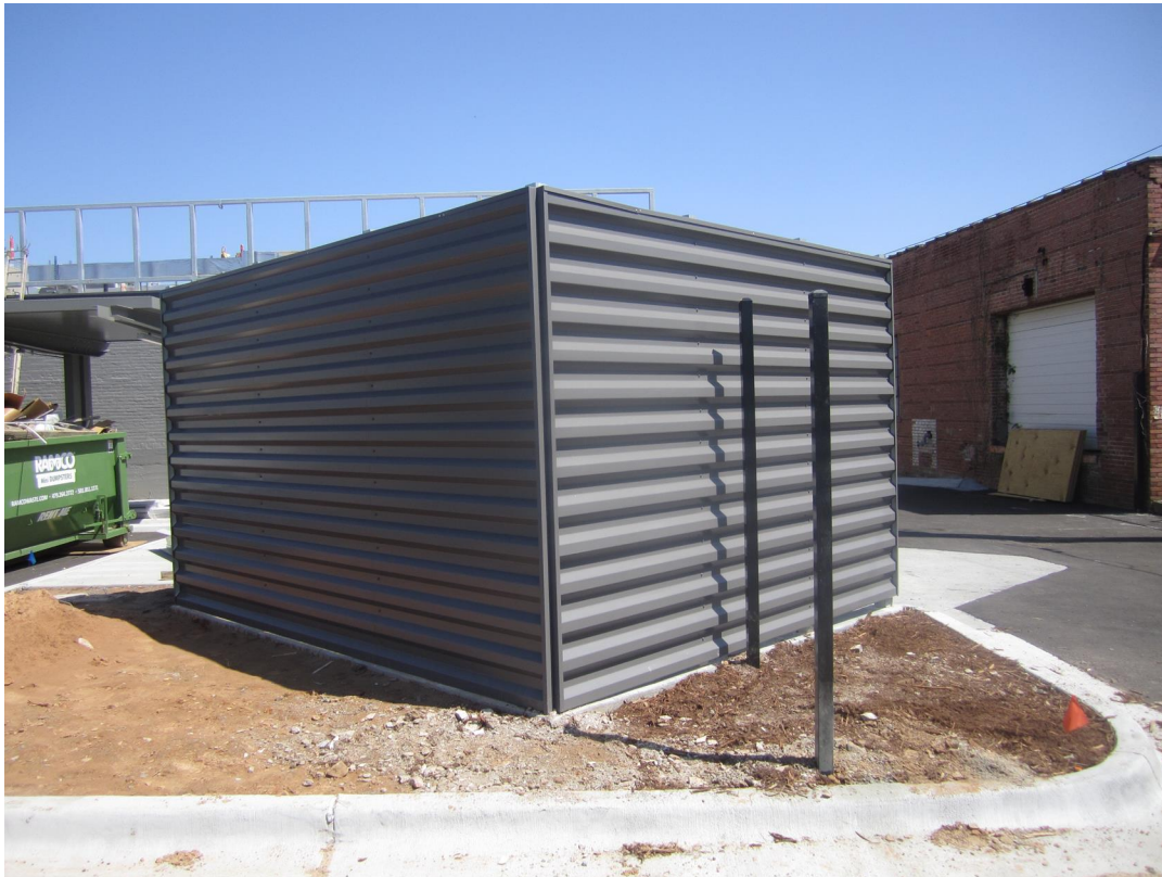
DUMPSTER ENCLOSURE IS COMPLETE
