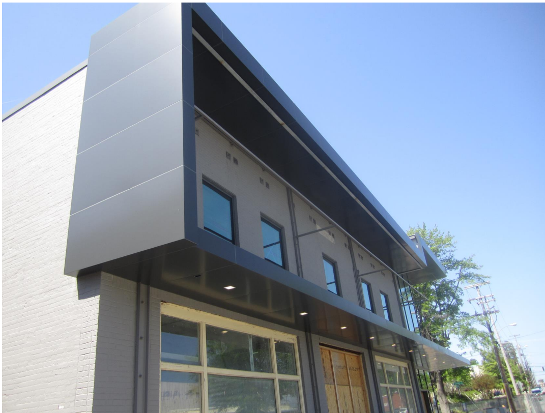
AMC PANELS @ NORTHEAST ELEVATION
