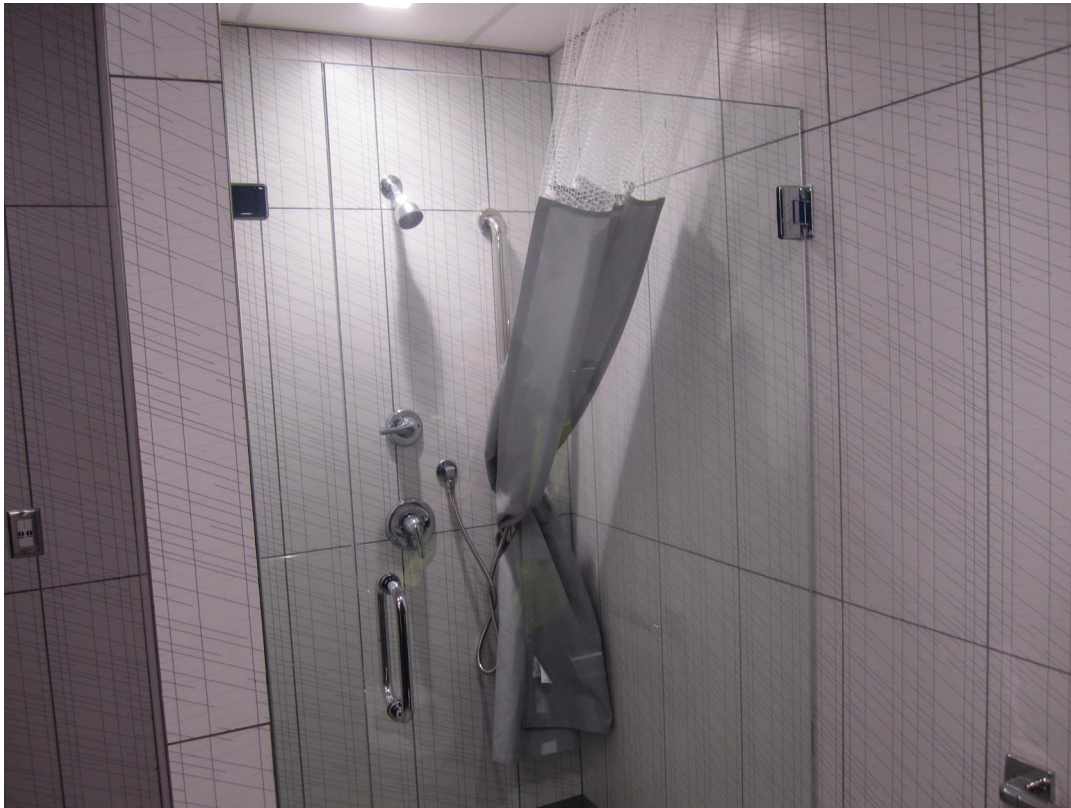
NEW GLASS SHOWER DOOR – CURTAIN & CURTAIN ROD TO BE REMOVED
