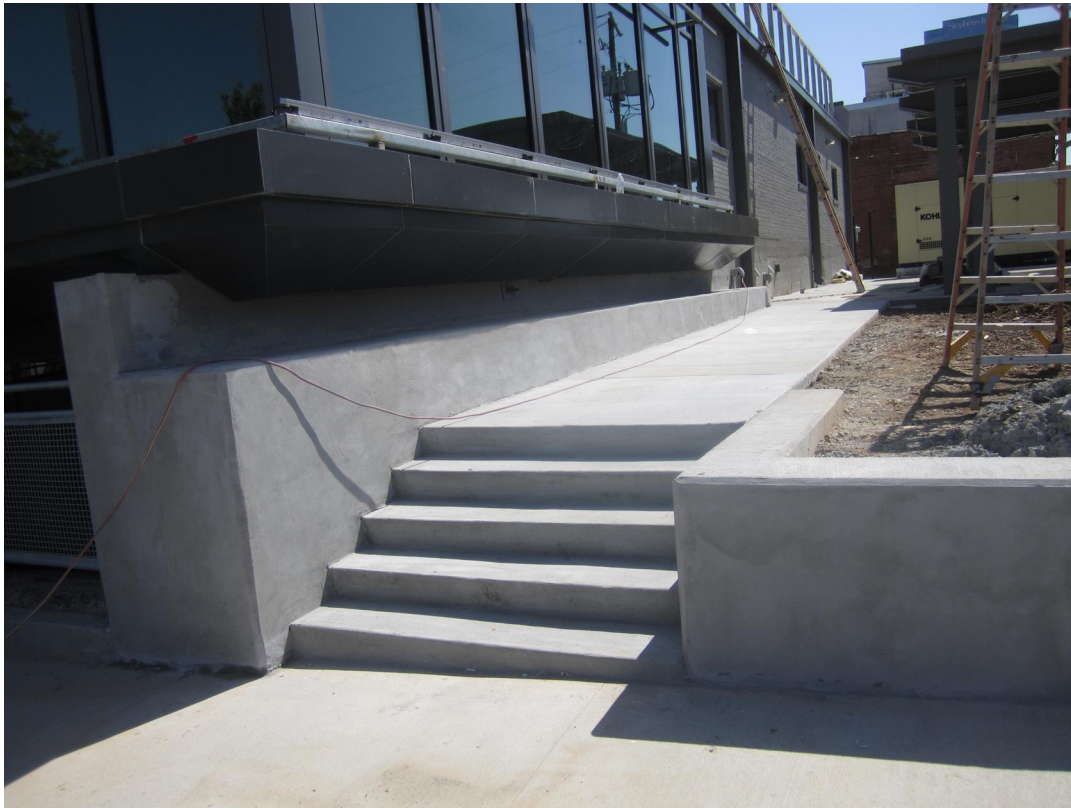
SOUTH SIDE WALK & LOW WALL IS FINISHED
