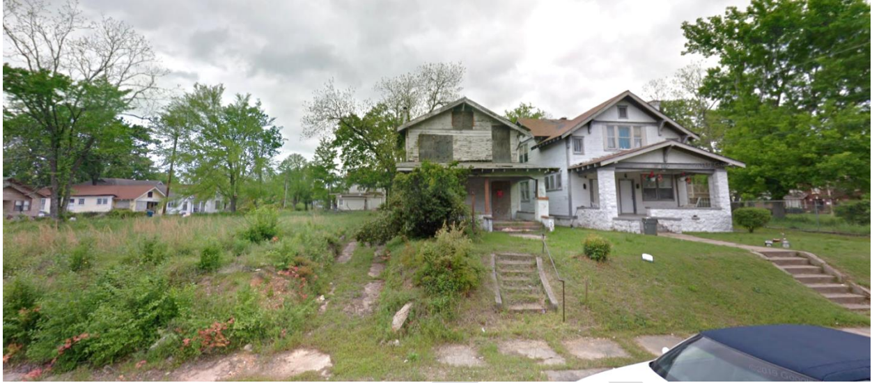
Figure 24. 2301-2309 Summit, before rehabilitation and infill construction, 2013.
