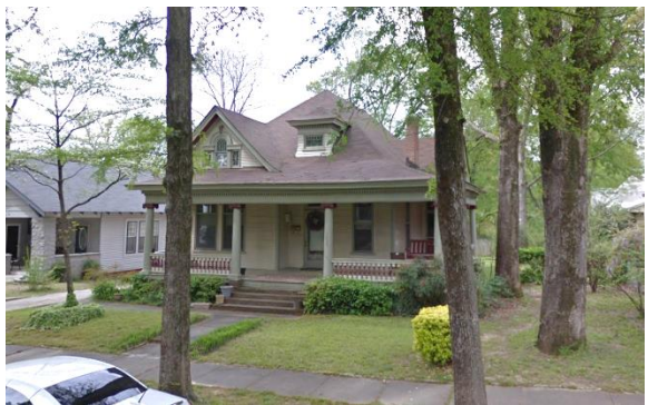
Figure 12. W.R. Stewart House at 1406 S. Summit, built in 1905 in the Colonial Revival style by architect Charles L. Thompson.
