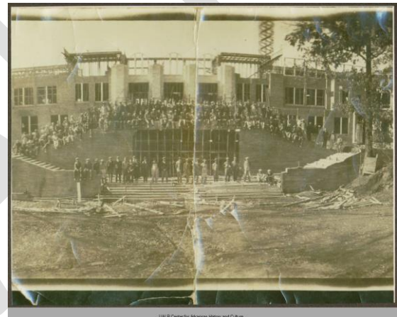
Figure 15. Central High during construction, c. 1927, courtesy of the Central Arkansas Library System.
