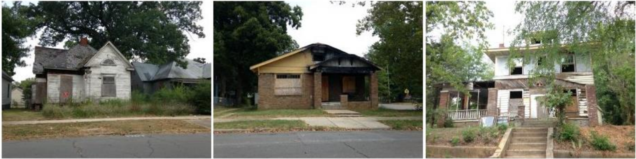
Figure 1. Vacant and deteriorating houses in the Central High Neighborhood Historic District, photos by Preserve Arkansas.
