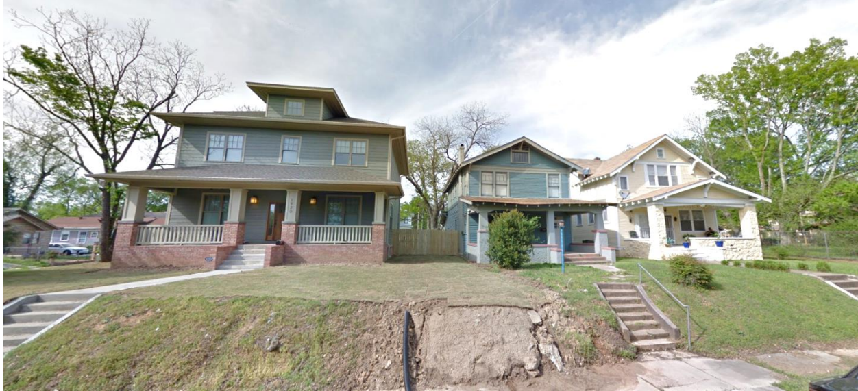
Figure 25. 2301-2309 Summit, after rehabilitation and compatible infill construction, 2019.
