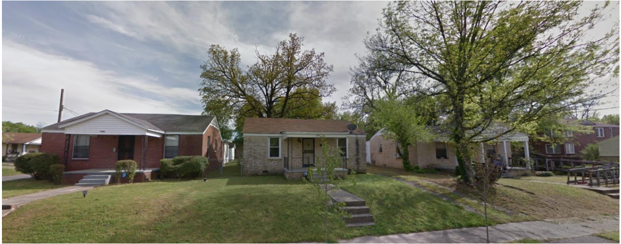
Figure 21. 1801, 1803, and 1805 W 18th Street all built in 1948 in the American Small House style.
