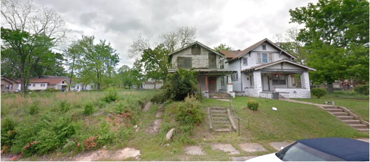
Figure 24. 2301-2309 Summit, before rehabilitation and infill construction, 2013.
