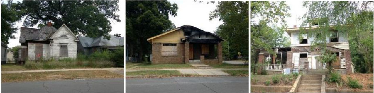
Figure 1. Vacant and deteriorating houses in the Central High School Neighborhood Historic District, photos by Preserve Arkansas.
