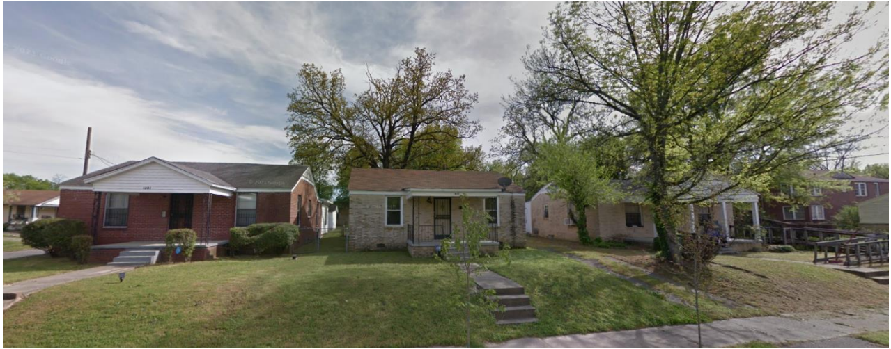
Figure 21. 1801, 1803, and 1805 W 18th Street all built in 1948 in the American Small House style.
