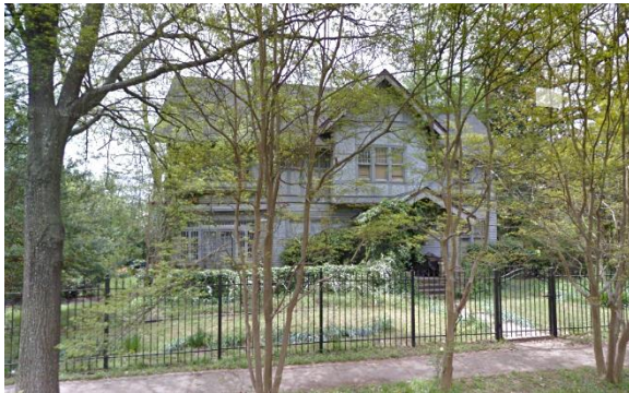
Figure 16. Warren Lenon House at 2005 W. 16th.
