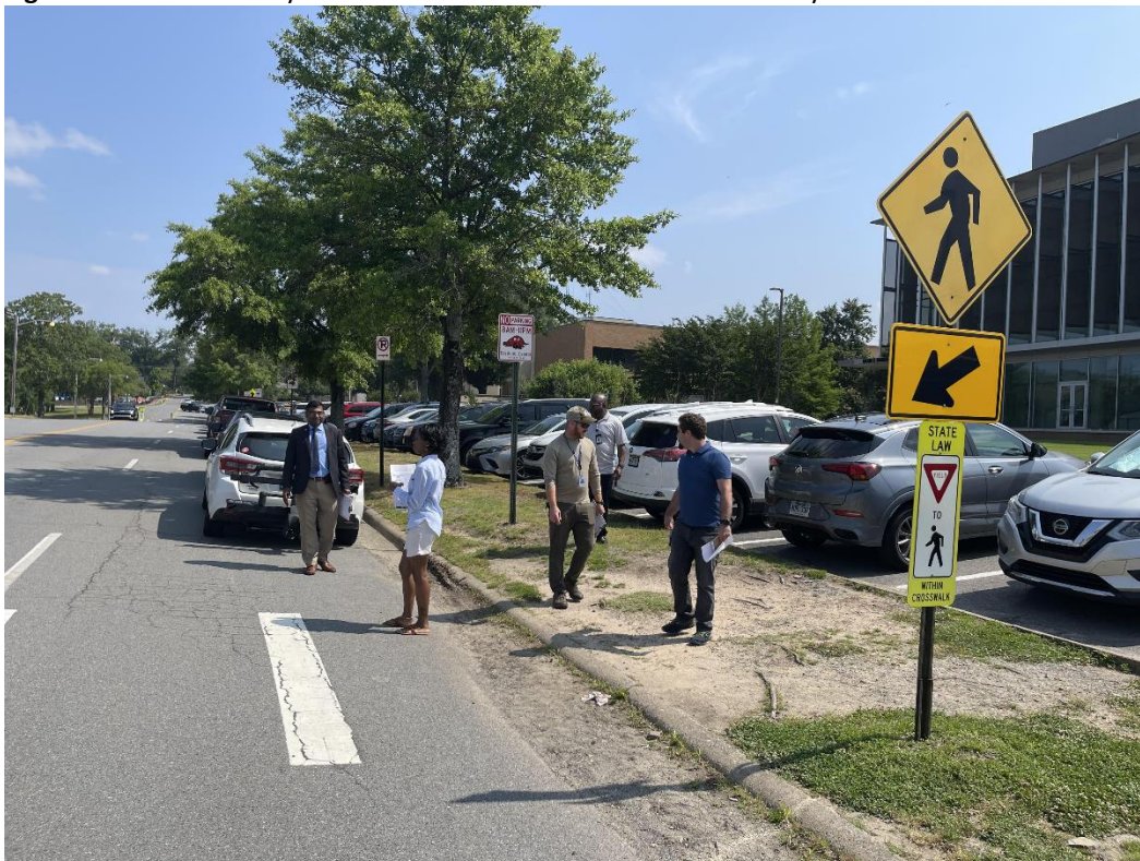
Figure A-5. One of two walk audit groups consider the Crosswalk 3 (Fig. 2), noting that 1) the white car is parked illegally close to the crosswalk and there is no infrastructure to stop this behavior, 2) there is no ramp at the end of the crosswalk, 3) there is no sidewalk at the end of the crosswalk, 4) signage at the side of the road and in the middle of the road is helpful, 5) hi-vis crosswalk markings are helpful, and 6) the crosswalk is not lit.
