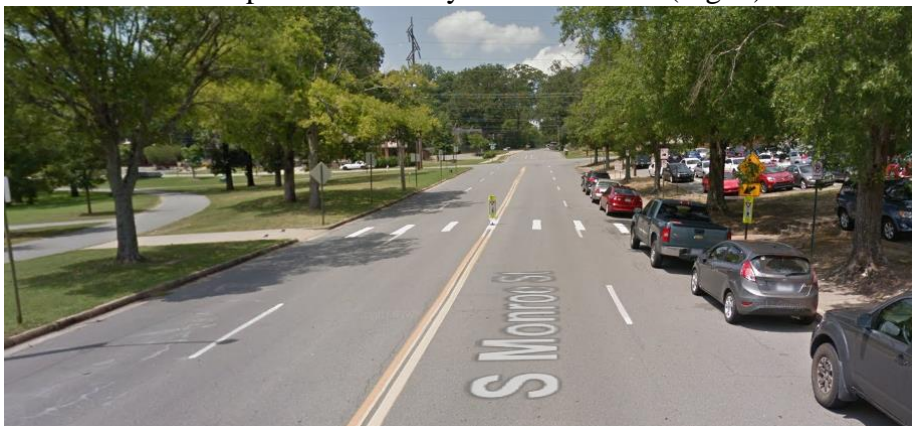
Figure 1. Crosswalks span four lanes of traffic with no refuge. Posted speed limit is 30mph, but cars drive faster due to street design speed. Parking is not allowed by crosswalk, but this signage is often ignored. Google Streetview, July 2017.
