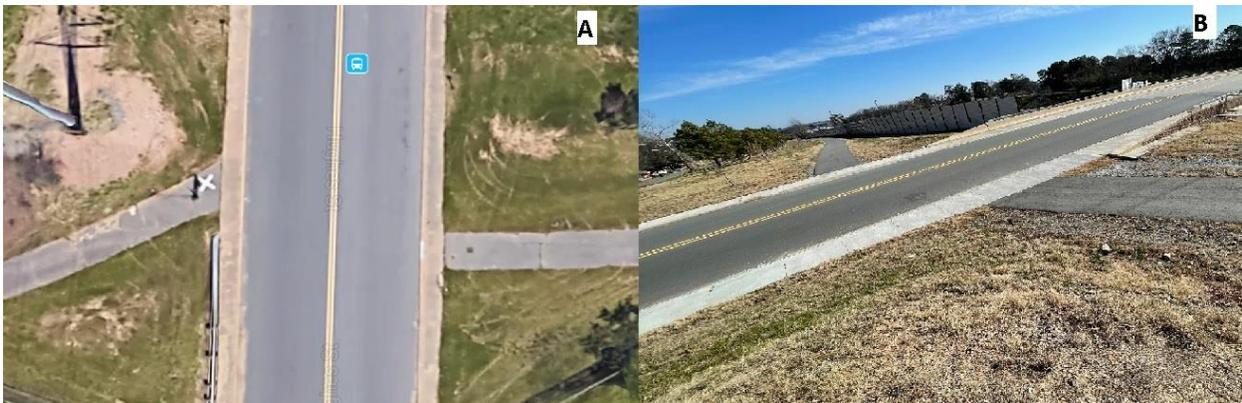
**Figure 6.** The I-630 Trail alignment A) before 2020 trail widening (Google maps) and B) after 2020 trail widening. ARDOT's 2020 work included realigning, rebuilding, and widening the trail, but ends in 6 in. high curbs on both sides of Hughes. The project needs a safe and convenient Hughes Street crossing.
