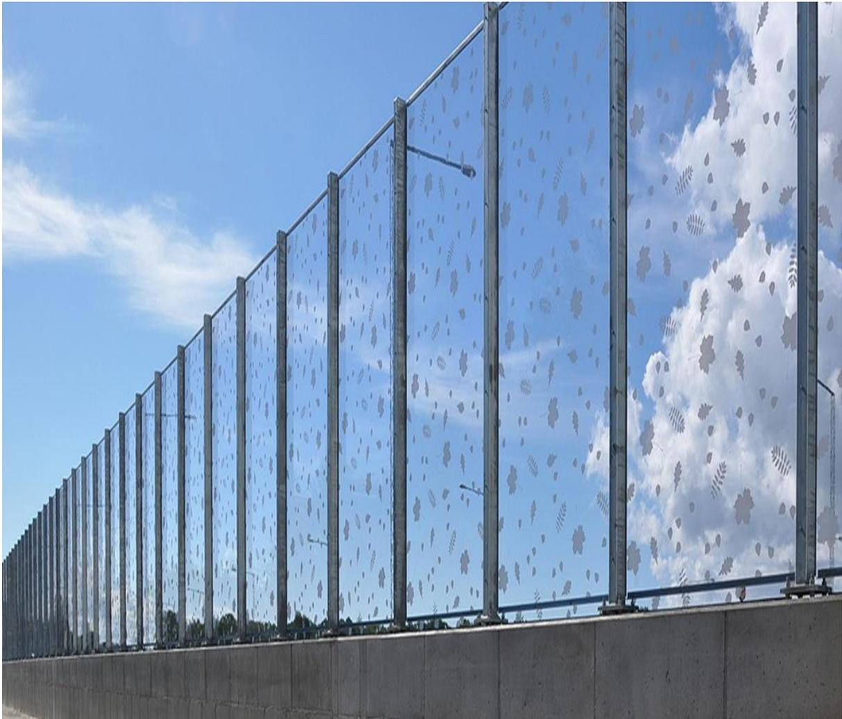
**Figure 10.** Acrylic sound barriers could be installed east of the Hughes crossing to increase sight triangles before the crossing.
