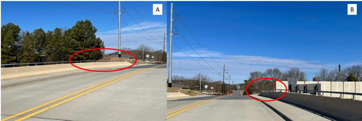
**Figure 9.** View from the Hughes northbound lane to the I-630 Trail entrances on the west side (A) and east side (B). Note that trail users in the crosswalk would be perfectly visible here (2 ft. high orange pail in (B) centerline), but users approaching the crosswalk would not be visible until shortly before reaching the sidewalk.
