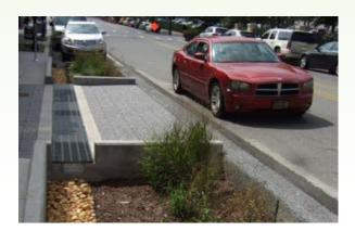
low impact development (LID) approach seeks to preserve open space and the natural water filtration systems through site design and features like rain gardens and bio-retention. The LID approach significantly increases retention of storm water and pollutants on site and generally does not threaten groundwater pollution. Porous pavements are extremely effective in filtering pollutants and reducing site runoff. Porous pavement has been reported to reduce runoff by up to 98 percent.
