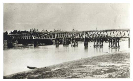
Baring Cross Bridge at Cross Street Constructed 1873, toll bridge added to top of bridge 1877
