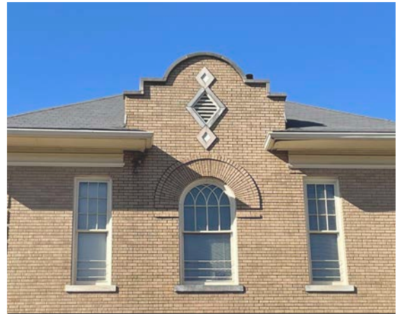
The parapet gable extending through the cornice is a significant roof feature of 314 E 8th St.
