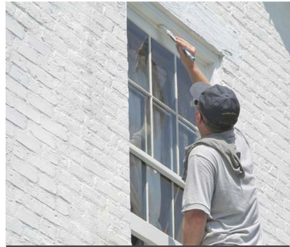
Scrape and repaint historic windows to protect wood from deterioration. © Indiana Landmarks
