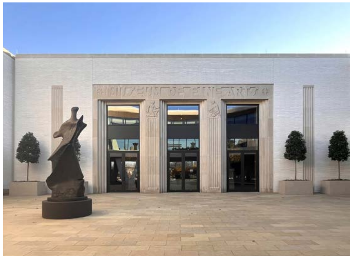
Institutional Building | Arkansas Museum of Fine Arts at 501 E. 9th St.
