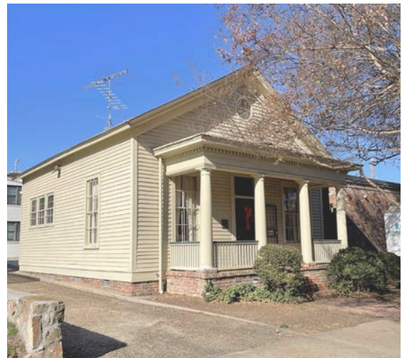
Preserve and maintain historic foundation materials that are in good condition, 610 S Rock St.
