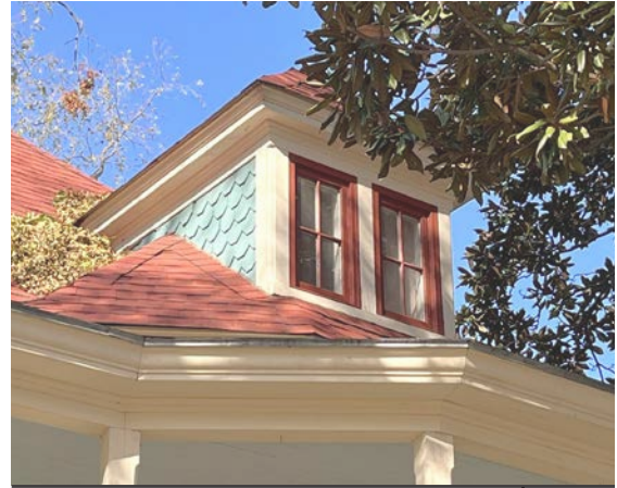
Well maintained dormer, 904 S Rock St.
