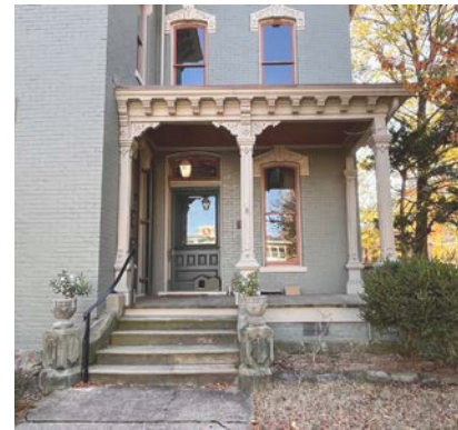
Porch handrails at Miller House, 523 E. 6th St.
