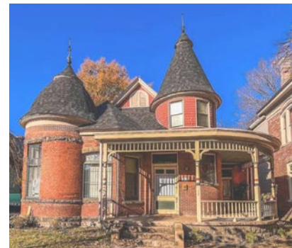
Historic stone porch foundation at 512 E 9th St.
