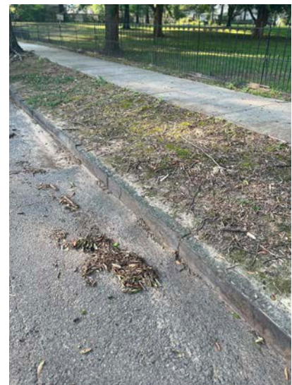
Concrete public sidewalks
