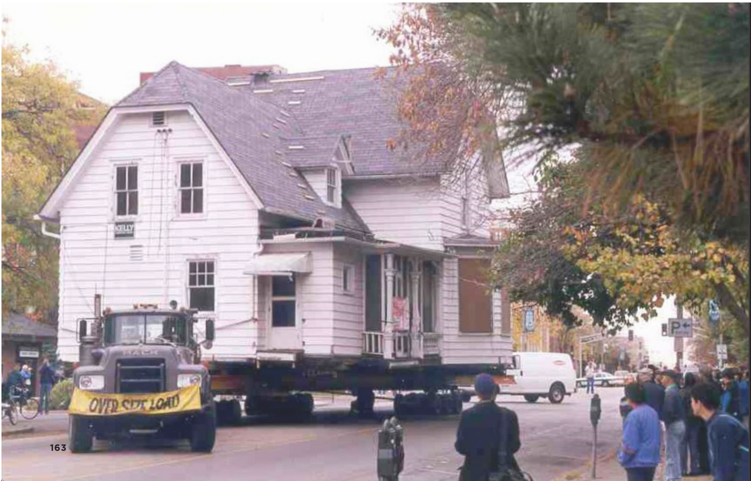
Relocation of a historic house. © Village of Oak Park, IL
