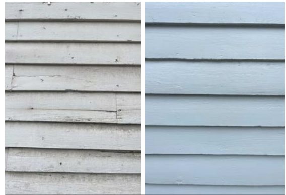
Whenever possible, repair rather than replace wood siding. If replacement is necessary, replace in-kind. Images above show wood siding before and after repair and paint.
