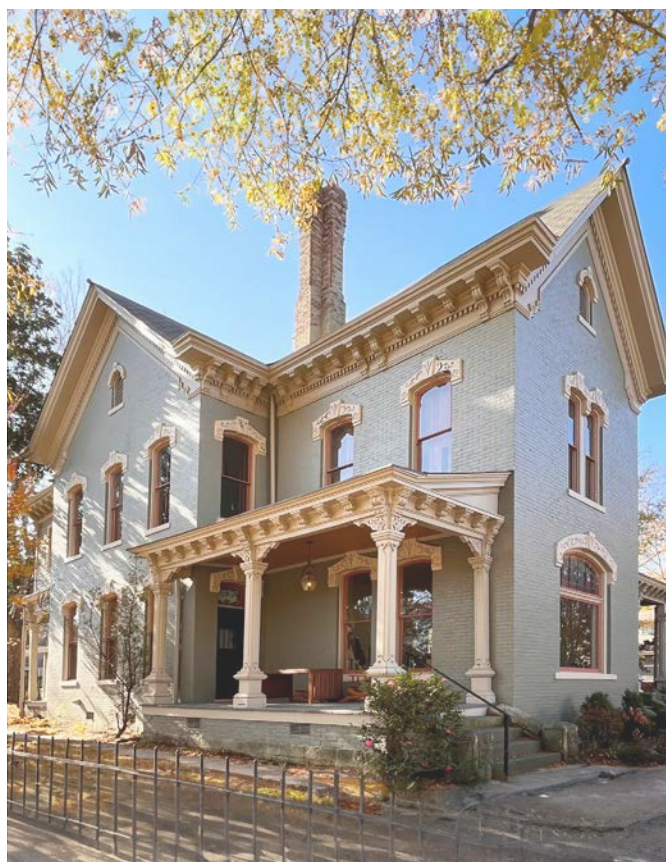
Wood architectural features of the Mills House, 523 E 6th St.
