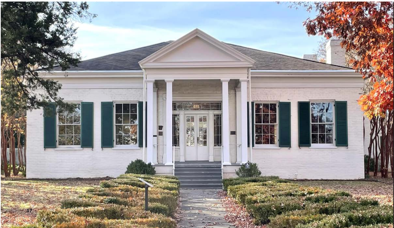
Curran Hall at 615 E Capitol Ave.
