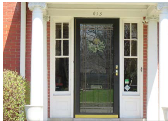
Add a storm door as a second full barrier against the elements.
