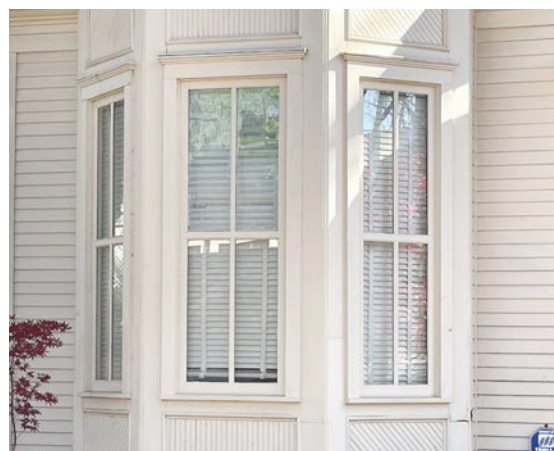
Maintain and repair window frames through repainting frames and replacing caulking, 609 S Rock St.
