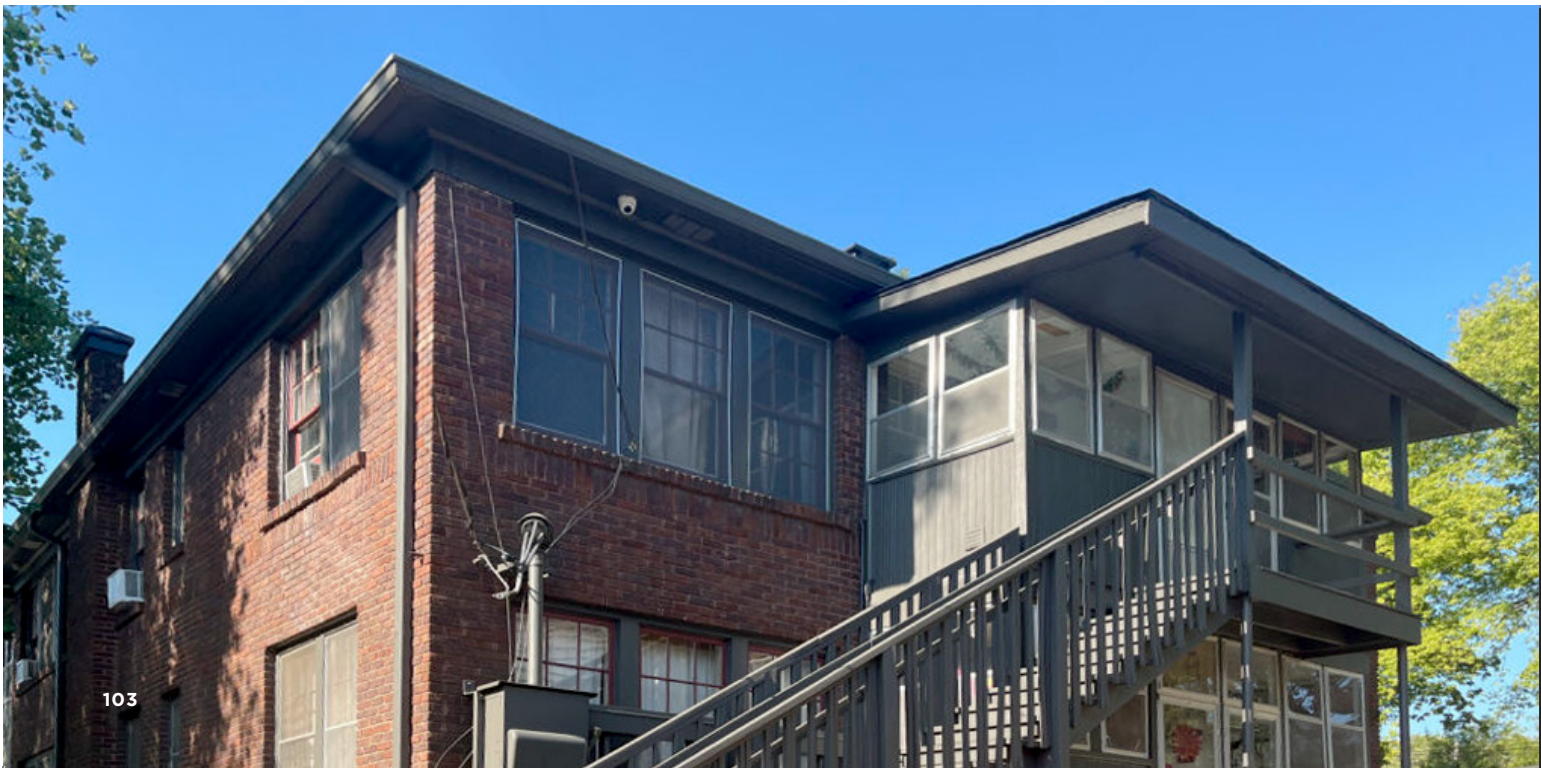
Place new staircases and fire escapes in areas minimally visible from the public right-of-way, 524 E. 6th St.
