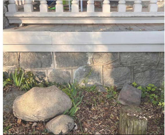
Do not paint masonry foundation surfaces unless historically painted, 514 E. 9th St.
