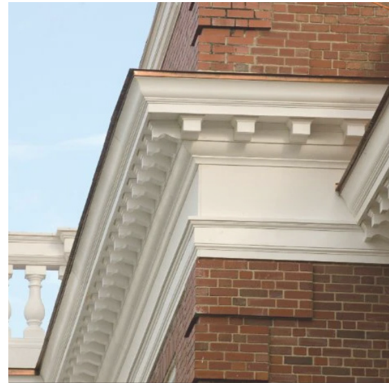
Replace original roof and cornice features using in-kind materials. © Worthington Millwork
