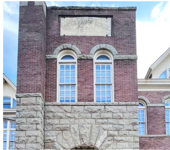
Upper story windows of Kramer School Lofts at 715 Sherman St.
