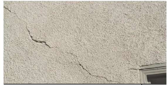
Do not ignore hairline cracks in stucco. Make sure to paint stucco to ensure its preservation.
