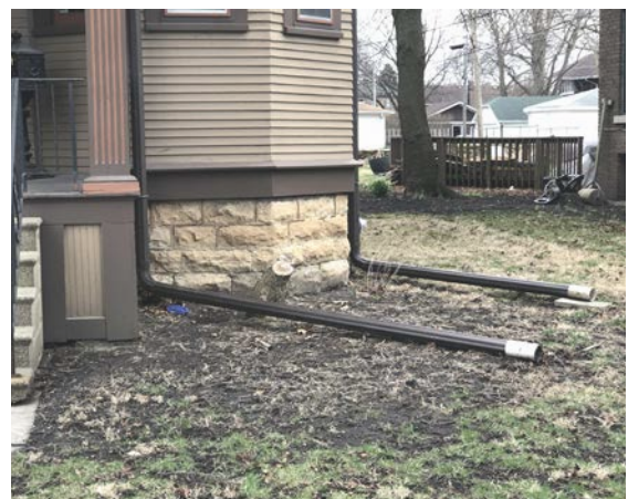
Locate downspouts away from significant architectural features to avoid water damage to the building.
