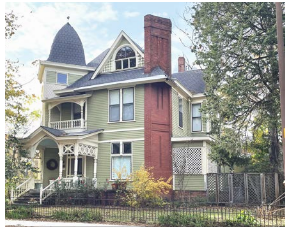
Anchor decorative features to prevent wind damage, Chisum House - 1320 Cumberland St.
