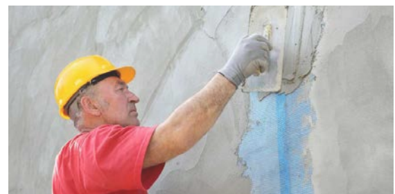
Do not use EIFS as a replacement to stucco. EIFS installations can lead to water retention and drainage issues. © JK Industries
