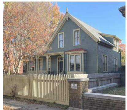
The house at 1011 S Scott St has a high-pitched roof.
