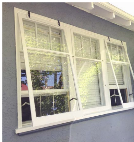
Add storm windows as a second barrier against the elements and air infiltration. © Spenser Works
