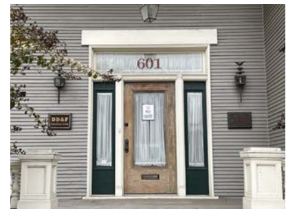
Historic door with sidelights and transom at 601 S Rock St., Nash House
