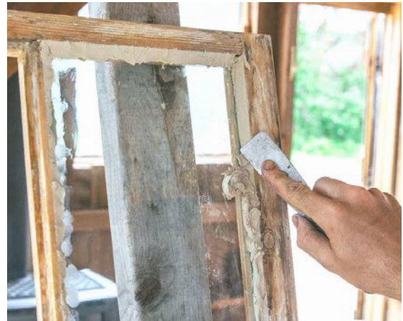
Remove damaged glazing and replace glazing putty. © Mortise and Tenon Magazine
