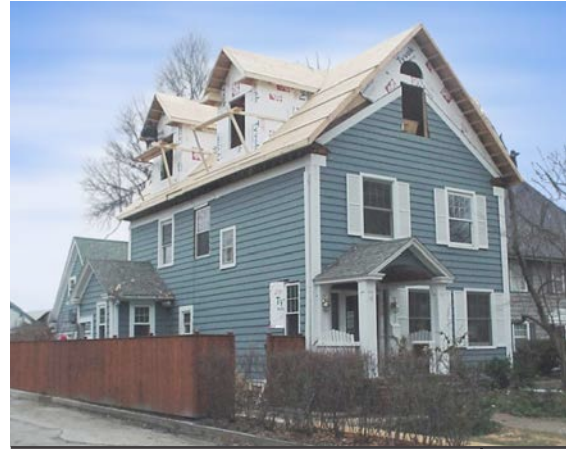
Do not alter or reconfigure the shape or slope of the main roof. © Village of Oak Park, IL
