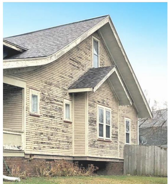
Use hand scrapers to remove peeling or blistered paint prior to repainting.
