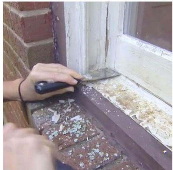
Carefully cut through the paint seal when reopening a window that is painted shut.
