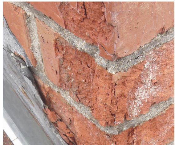
Do not use portland cement as a type of mortar, as this will cause spalling. © Hudson Valley Chimney
