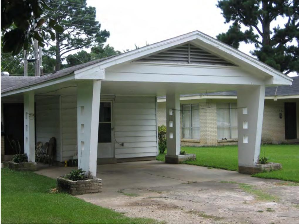
Figure 95: Detail of the slanted concrete carport pylons at 7219 Azalea Drive.
