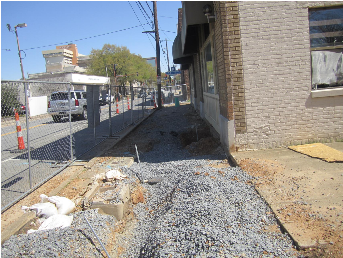
CORNER OF GAINES & MARKHAM STORM DRAIN
