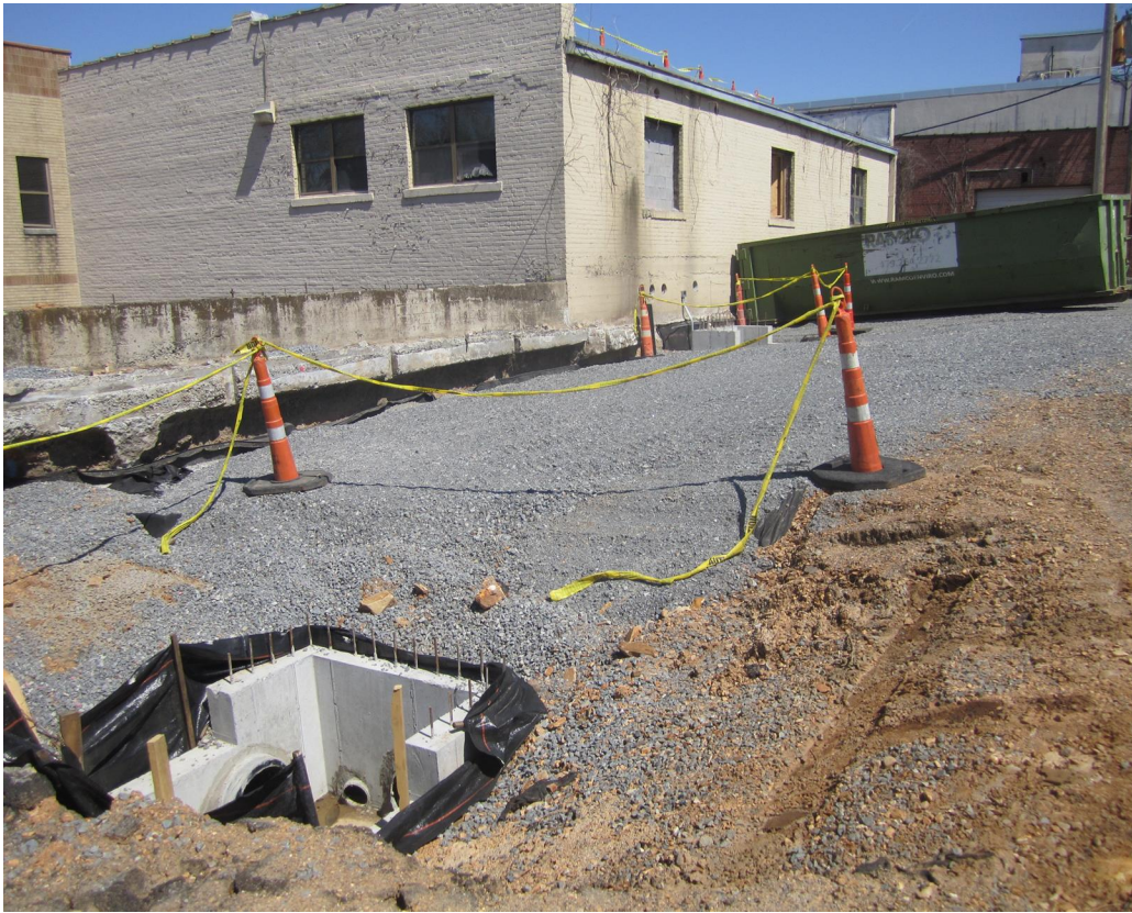
SOUTH WALL – BACKFILLING
