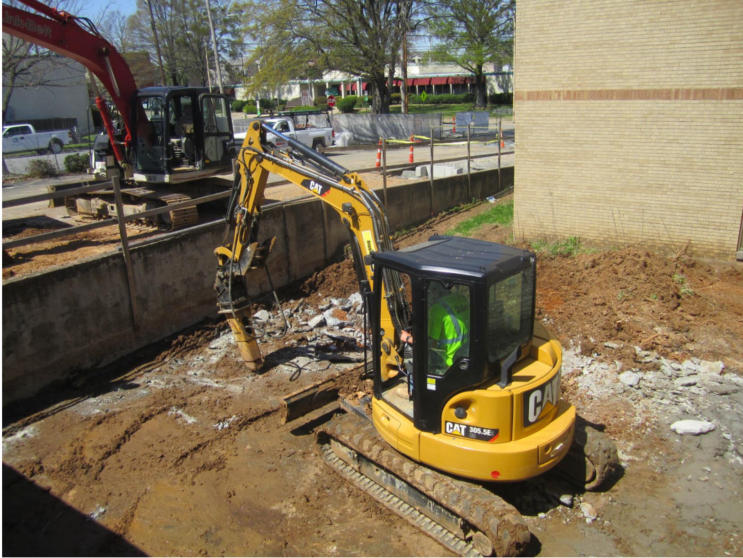
DEMOLITION OF EXISTING 8" CONCRETE SLAB
