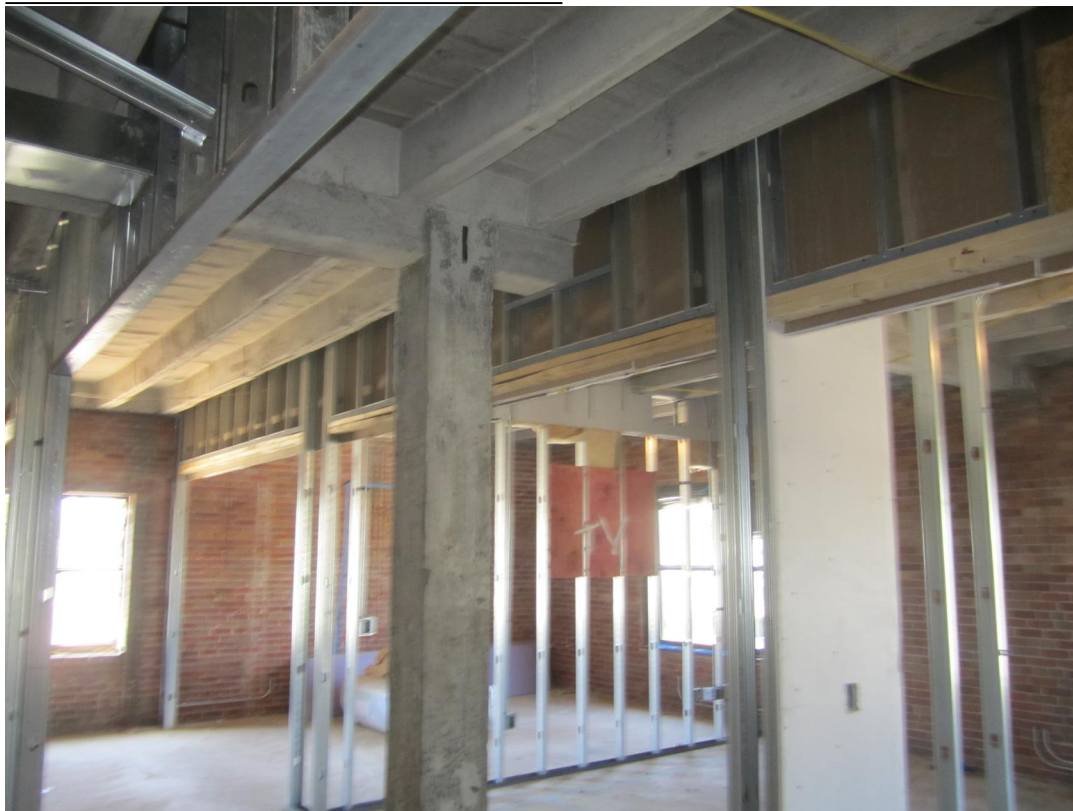
2 ND FLOOR BLOCKING AT TOILET AREA
