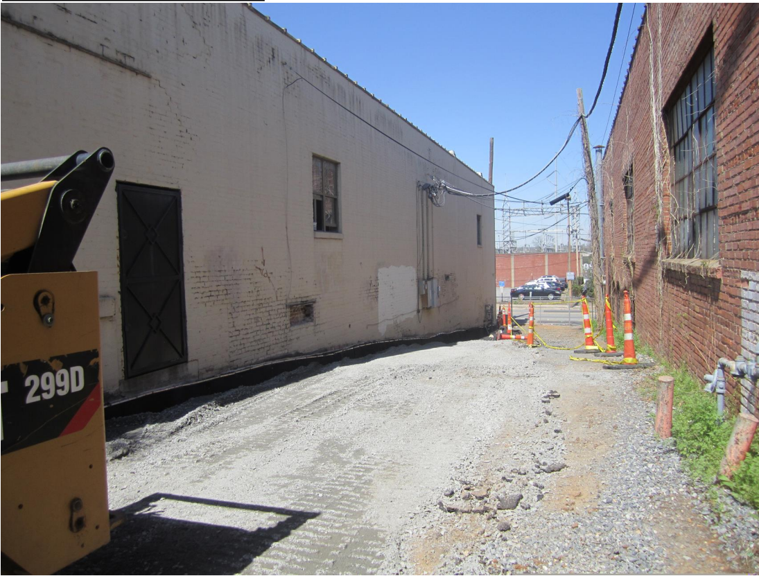
EAST WALL BACKFILLING
