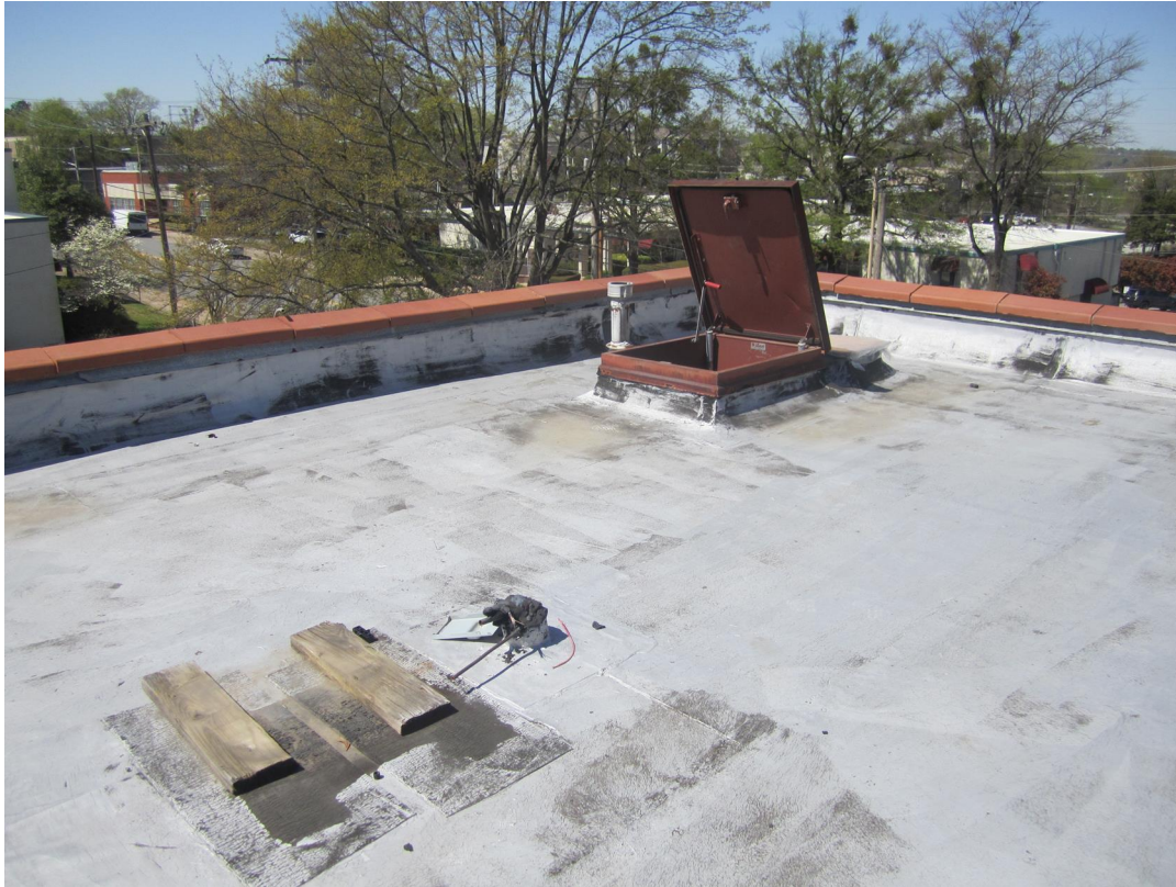
UPPER ROOF LOOKING NORTHWEST – EXISTING HVAC UNITS REMOVED
