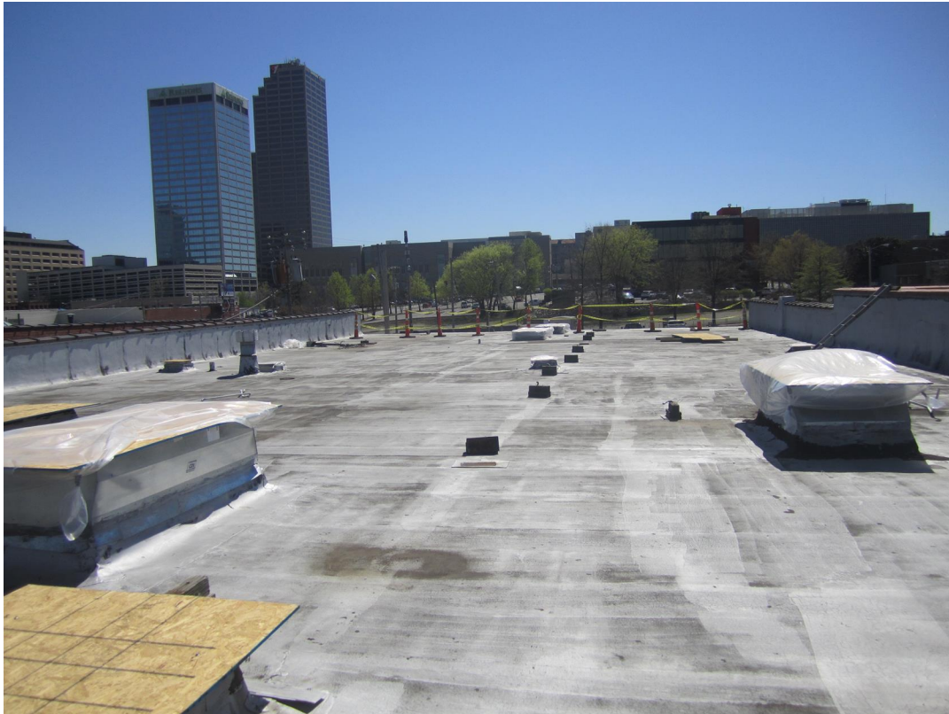
LOWER ROOF LOOKING SOUTH – EXISTING ROOF TOP UNITS REMOVED & NEW CURB INSTALLATION
