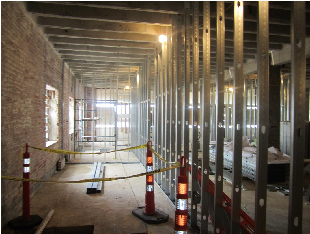
1 ST FLOOR METAL STUD INSTALLATION
